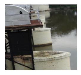
The movement of the counterweights creating stress at the column may be minimized by providing additional structural support between the pier top and the edge of the Chequered plate platform as shown in the picture.
