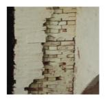
• The pointing mortars may have been removed by the impact of flood waters entering the widened cracks.
