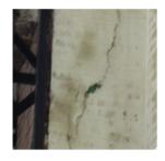
• The process of crack initiation, the subsequent widening of the crack and the later damage to brick joint pointing have occurred over a prolonged period of time and the process has been long drawn out.
